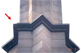
Fig. 7: Close-up view of the lightning damaged section of the minaret (arrowed).
