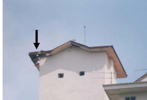
Figure 6: A photograph of the other Setapak Ria apartment building showing a different French made ESE air terminal and the stricken point.
