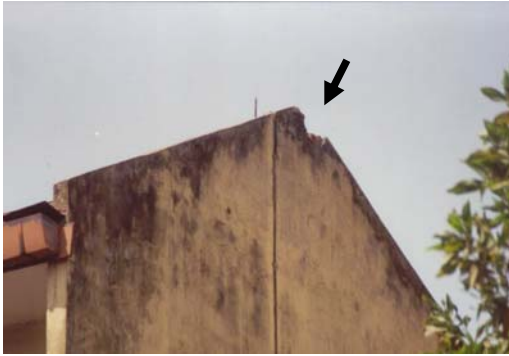
Figure 12: A close-up photograph of another apartment block showing the stricken point and the Franklin rod beside it. For effective protection, the rod must be positioned right on the ridge ends and similar high risk locations.
