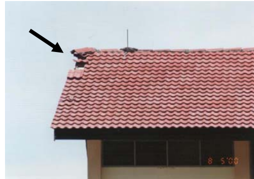
Figure 9: Photograph of a stricken point at the gable roof ridge end. The Franklin rod should have been installed right on top of the ridge end instead of about 1m away from it.
