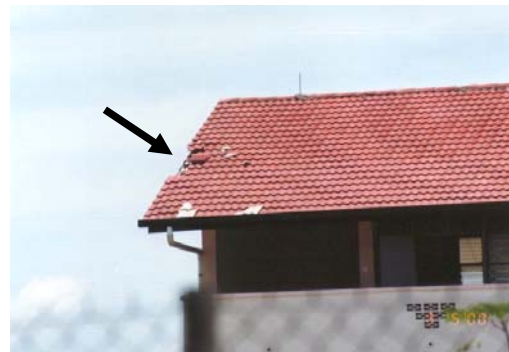
Figure 10: Photograph of a stricken point on the slanting edge of the gable roof. The air terminal conductor should also be installed on the edges of the gable roof.
