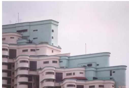
Figure 7: Photograph of the Villa Putri apartment building showing the two Australian made ESE air terminals installed on the split-level roofs.
